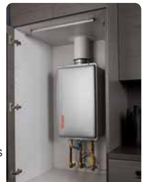
Example of an HDi200 installed in a cupboard - Rinnai Auckland showroom
